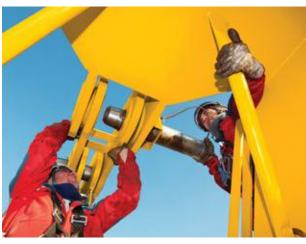
Fitting and pinning the jib requires only one pin at the top.
